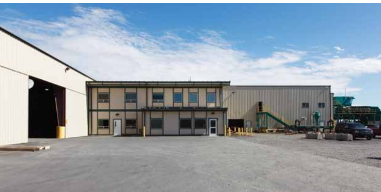
Upper Columbia Mill – Boardman, Oregon, USA
